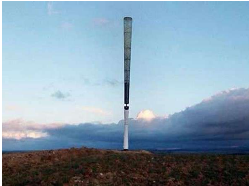
Fig. 2: Bladeless wind turbine ( Courtesy : Urja Daily)
